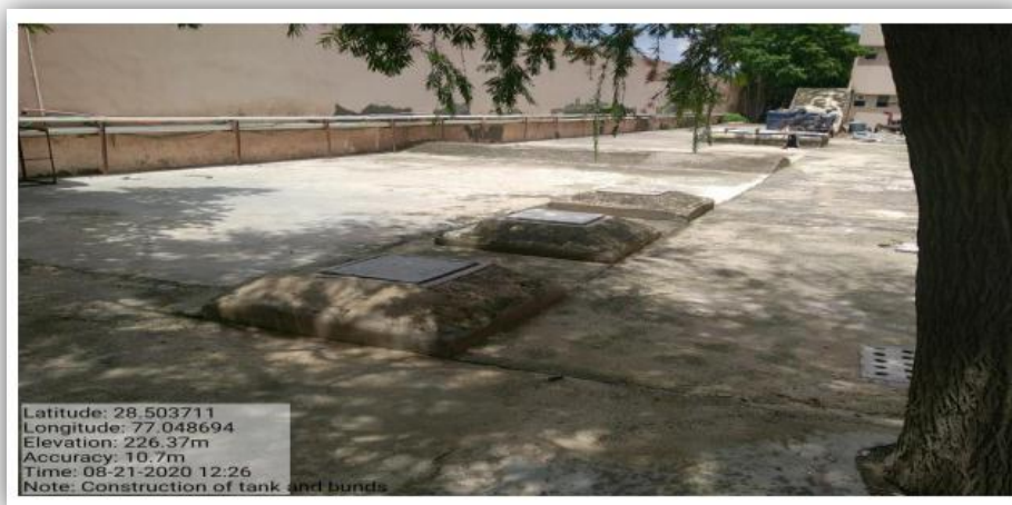
Figure 2: Construction of tanks & bunds
